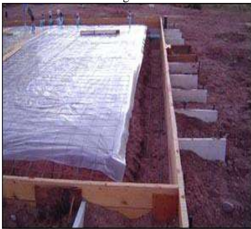
Fig: Plastic sheet covering of concrete
