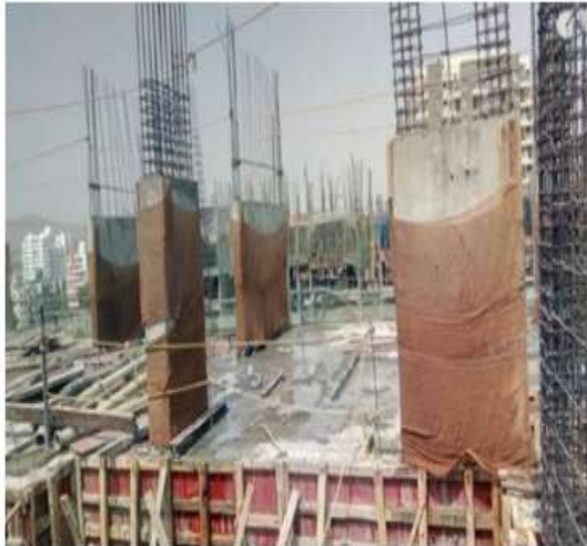
Fig: wet covering by hessian cloth
